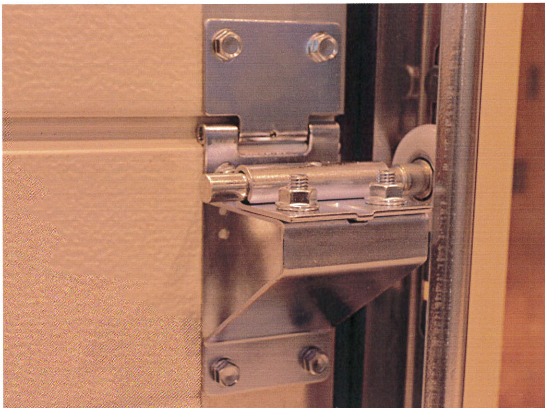
Figure 3. Side hinge, slide and roller.
