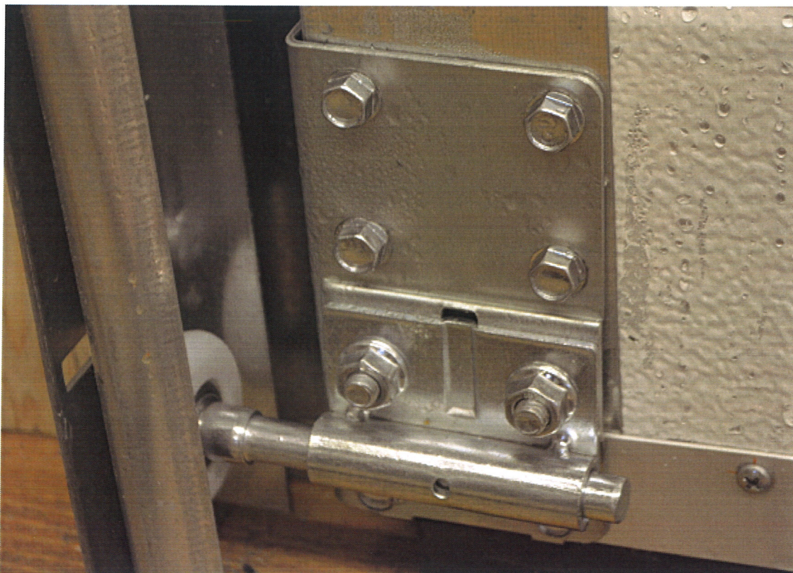
Figure 4. The bottom bracket.
