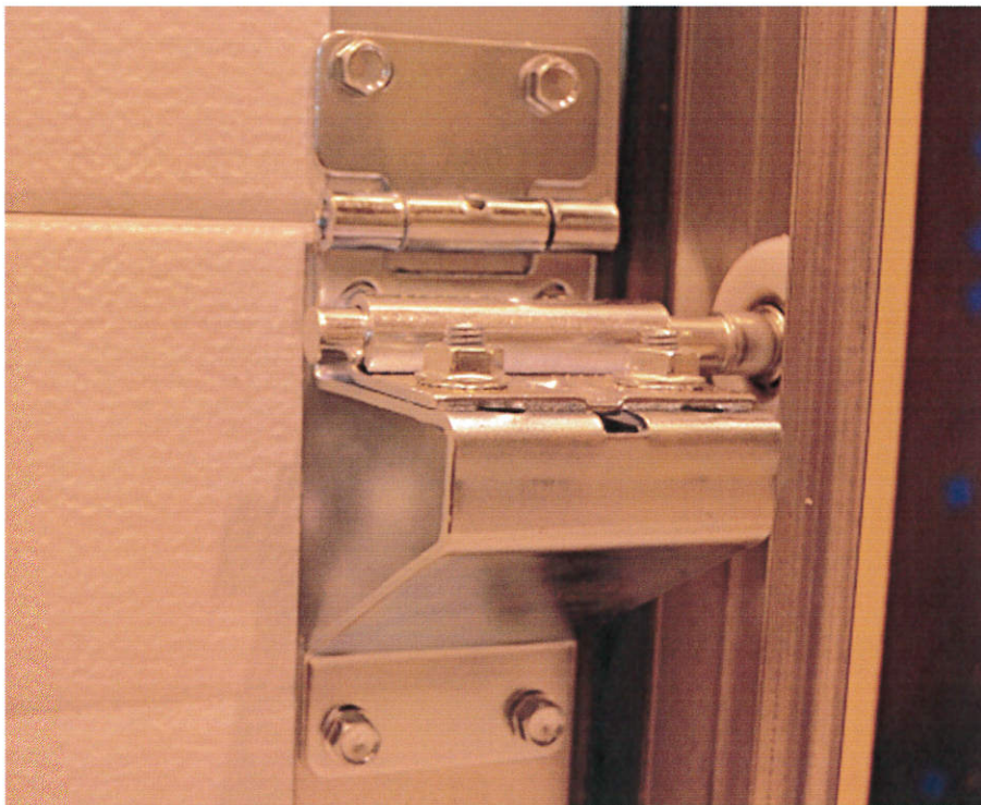
Figure 3. Side hinge, slide and roller.
