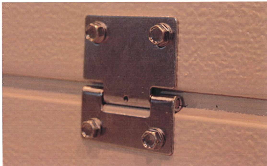
Figure 4. Intermediate hinge.
